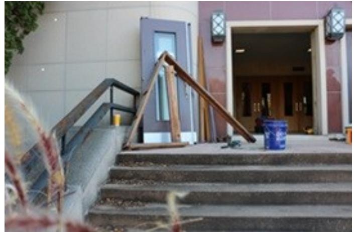
New 16th Street doors - installation in progress
