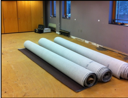
Rolls of carpet await installation in chapel
