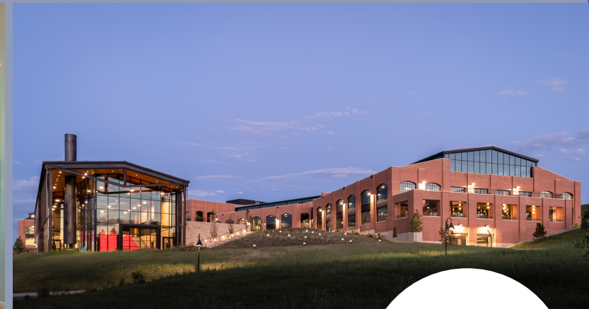
Partners Group HQ, Broomfield New 4-building campus
