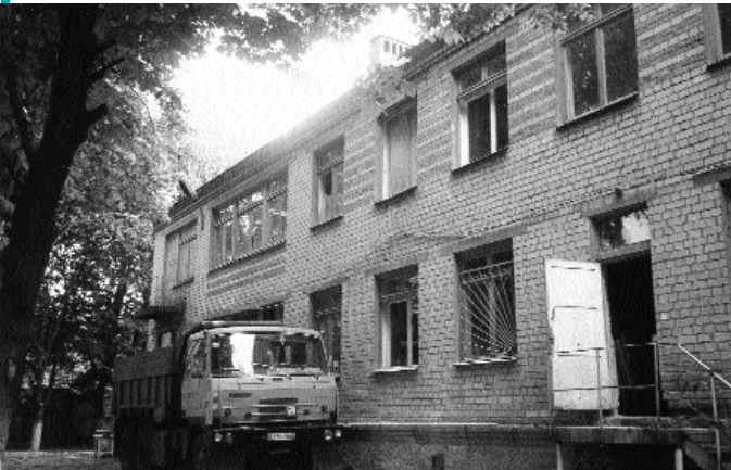
Renovation and construction taking place at GJARN's new medical center site.
