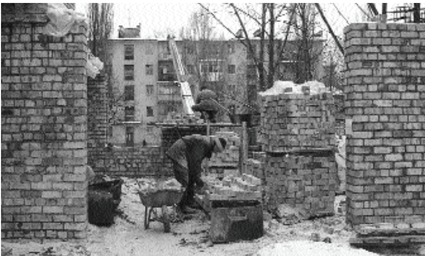
Construction on American Jewish Medical Center continues, even in frigid weather.
